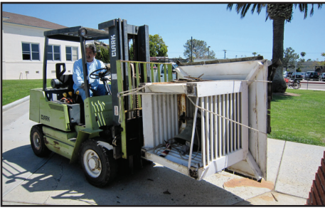
San Dieguito's faculty, staff and students were shocked when a wrecking crew showed up on campus to demolish our bell tower.
