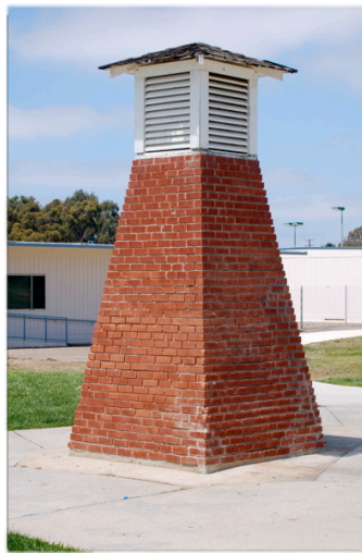
The bell tower as it appears today. The louvers were installed in 1987 to protect the new bell from vandalism.
